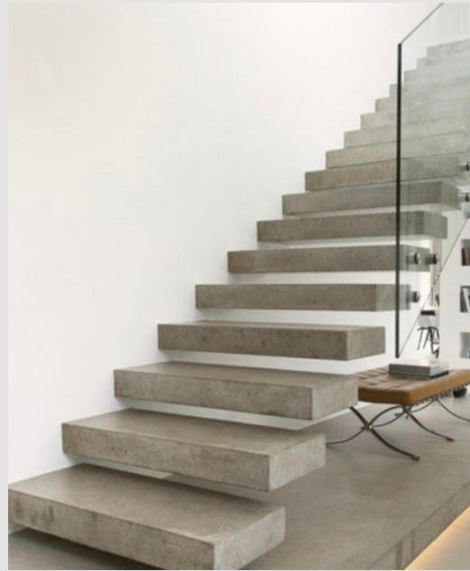
Floating Stairs with frame-less glass
