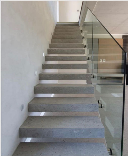
Floating Stairs with frame-less glass
